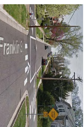
Raised intersections are essentially speed humps that fill the area between the four corners
