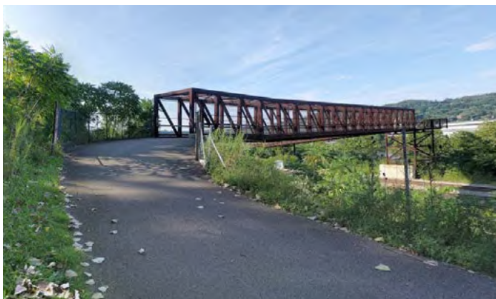
This trail bridge for the Great Allegheny Passage crosses a multi-track railroad corridor in West Mifflin, PA. Its length, including approach ramps and the bridge span, is approximately 1,100 feet. Its cost was $9 million.
