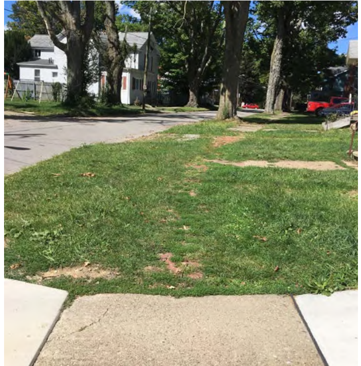
Some older brick sidewalks are overgrown with lawn, making them hard to see and rough to traverse.
