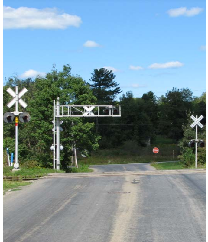
Active railroad crossing at Gates Street
