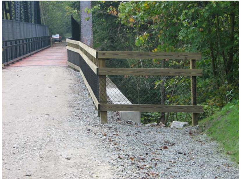
Figure 4.11 Example of a Timber Approach Railing at Bridge
