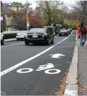
Example of Bike Lane at sidewalk
