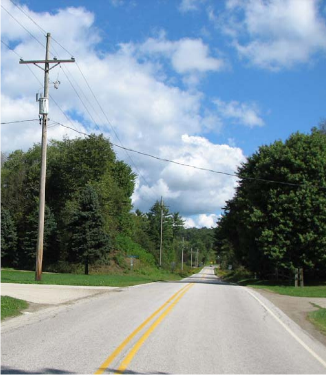
Former ROW Crossing at SR 89 (structure missing)
