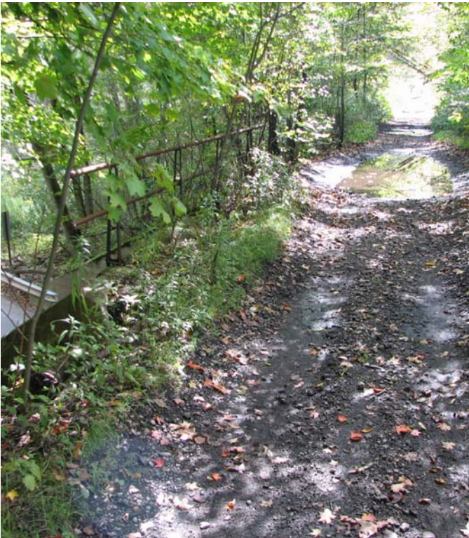
Former ROW Crossing over Concord Road
