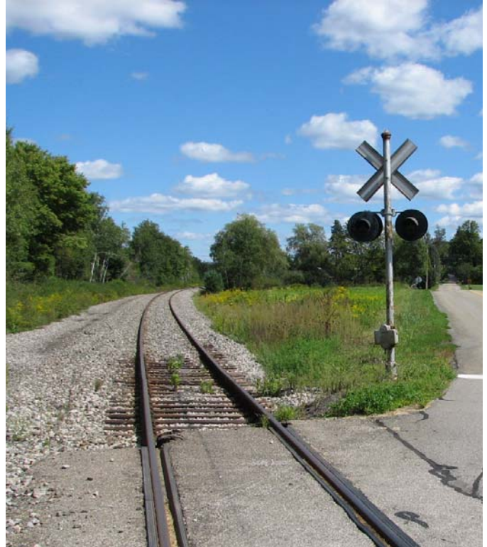
Lovell Road Active Railroad Crossing
