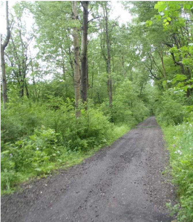
Typical Corridor in Segment 1
