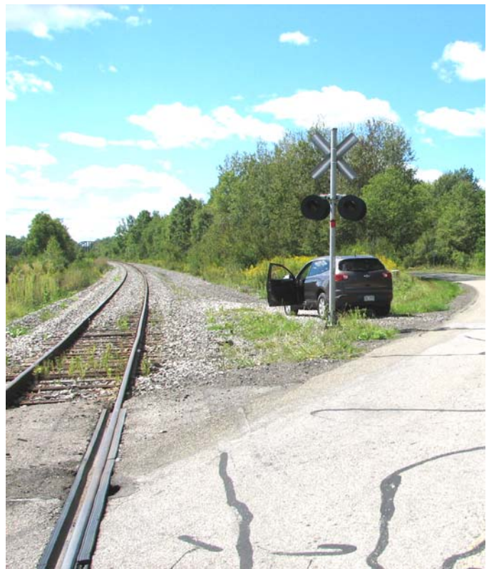
Lovell Road Active Railroad Crossing
